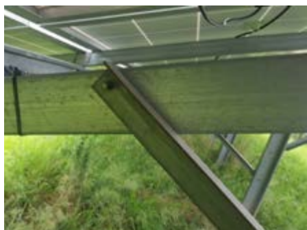
7750 kWp in Hachenburg, Germany
