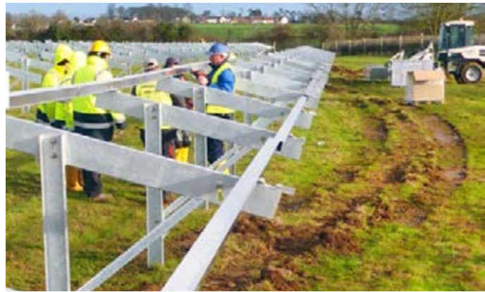
Ramming of the support profiles.
